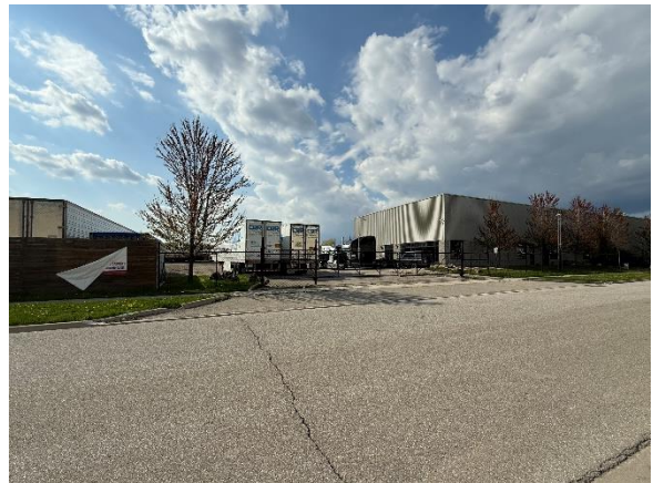
SUBJECT BUILDING EXTERIOR – SITE ACCESS FROM ADVANCE ROAD
