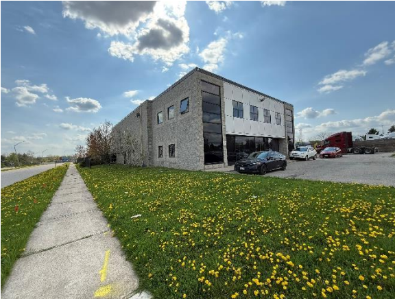
SUBJECT BUILDING EXTERIOR – SOUTHERN EXPOSURE OF BUILDING
