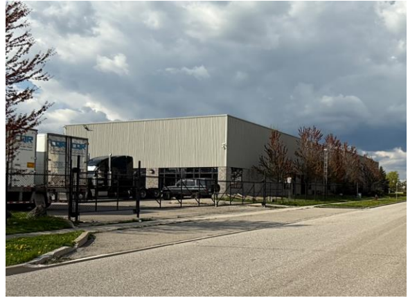
SUBJECT BUILDING EXTERIOR – SOUTHERN EXPOSURE OF BUILDING
