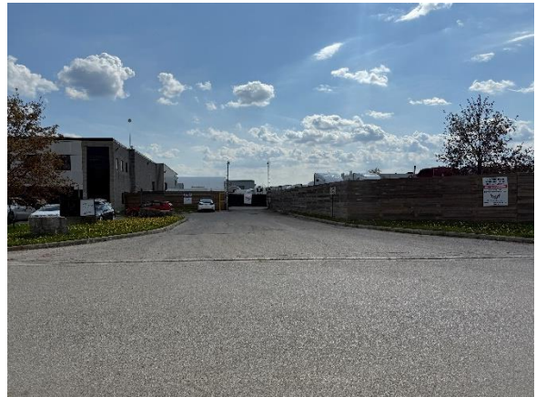
SUBJECT BUILDING EXTERIOR – SITE ACCESS FROM PROGRESS COURT
