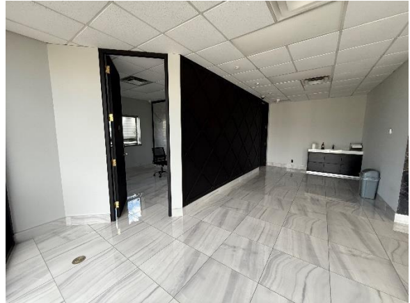
SUBJECT BUILDING INTERIOR – GROUND FLOOR OFFICE AREA
