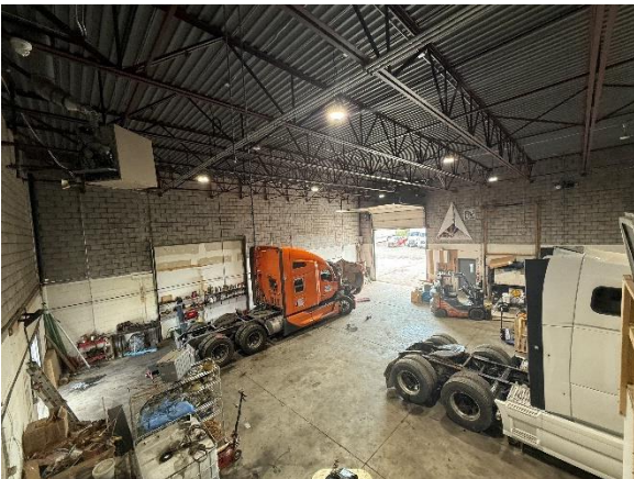
SUBJECT BUILDING INTERIOR – INDUSTRIAL AREA, EASTERN PORTION
