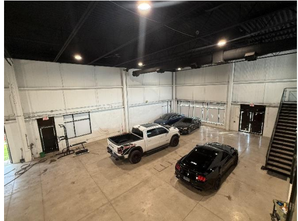
SUBJECT BUILDING INTERIOR – INDUSTRIAL AREA, WESTERN PORTION
