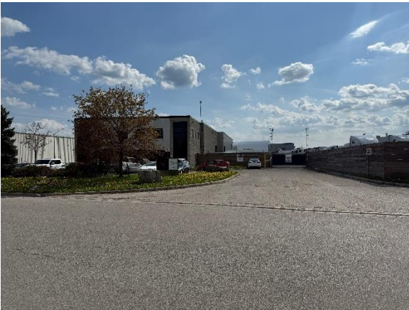
SUBJECT BUILDING EXTERIOR – PROGRESS COURT STREET FRONT
