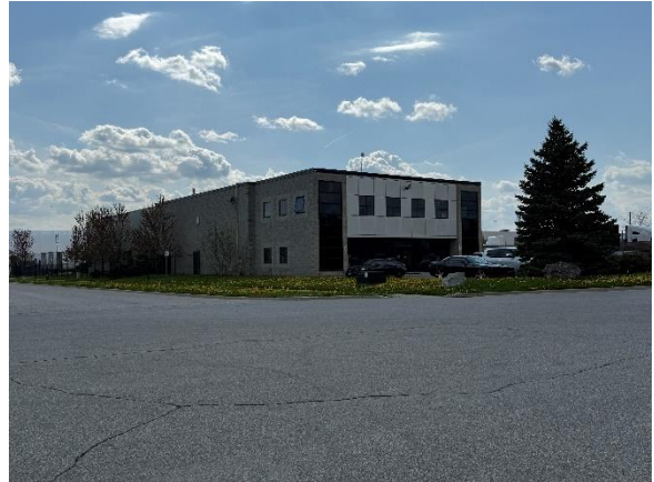
SUBJECT BUILDING EXTERIOR – PROGRESS COURT STREET FRONT
