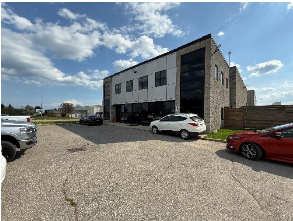
SUBJECT BUILDING EXTERIOR – STREET FRONT OFFICE AREA, MAIN ENTRANCE
