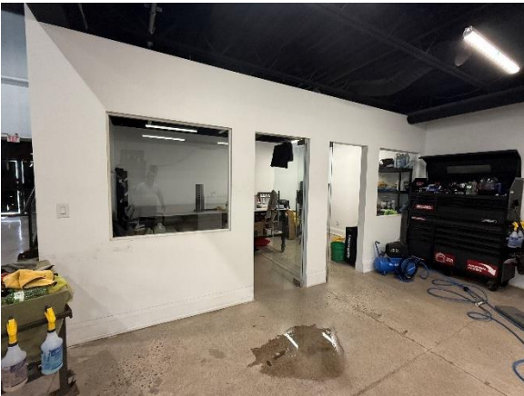
SUBJECT BUILDING INTERIOR – INDUSTRIAL AREA, WESTERN PORTION
