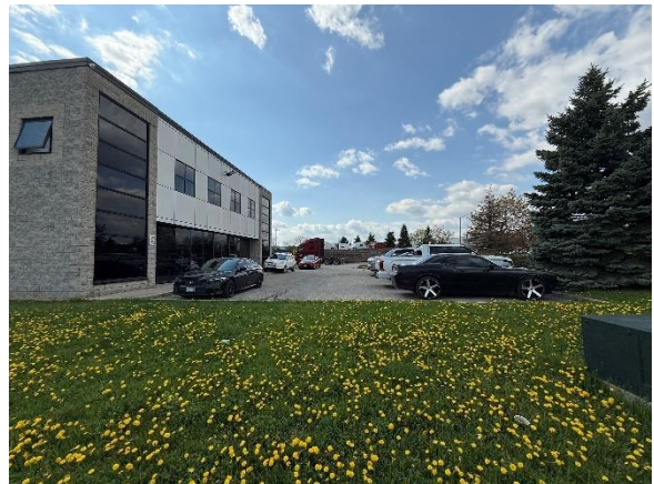
SUBJECT BUILDING EXTERIOR – STREET FRONT SURFACE PARKING AREA
