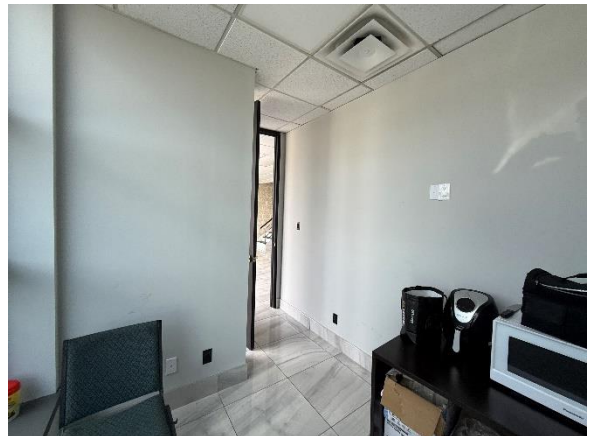
SUBJECT BUILDING INTERIOR – GROUND FLOOR OFFICE AREA
