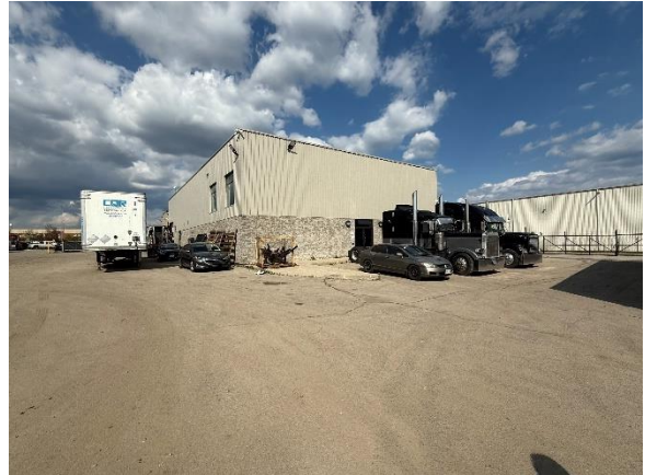
SUBJECT BUILDING EXTERIOR – WESTERN EXPOSURE OF BUILDING, REAR
