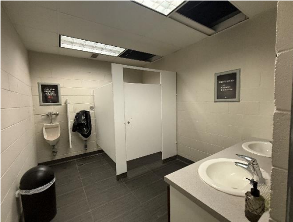
SUBJECT BUILDING INTERIOR – INDUSTRIAL AREA, WESTERN PORTION
