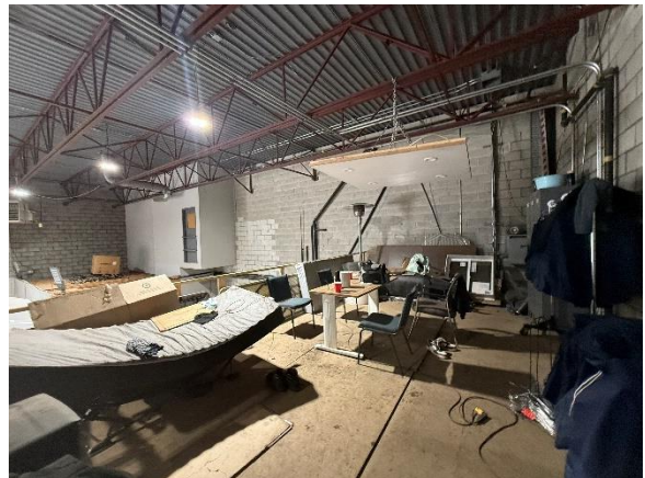
SUBJECT BUILDING INTERIOR – INDUSTRIAL AREA, EASTERN PORTION
