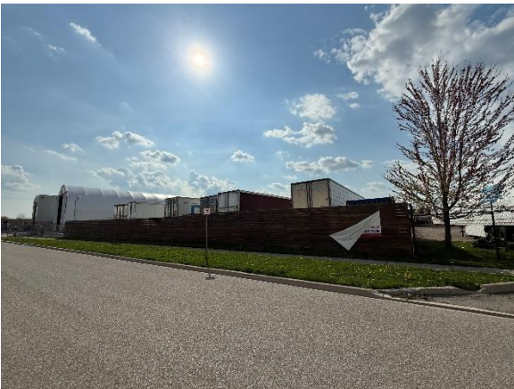
SUBJECT BUILDING EXTERIOR – REAR FENCED YARD AREA, VIEW FROM ADVANCE ROAD
